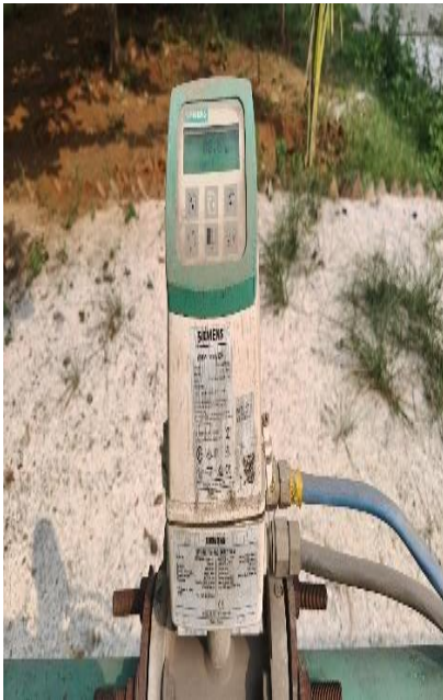
FOR COOLING PURPOSE
