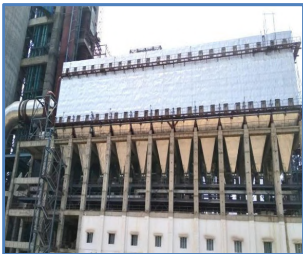
RABH for Kiln & Raw Mill
