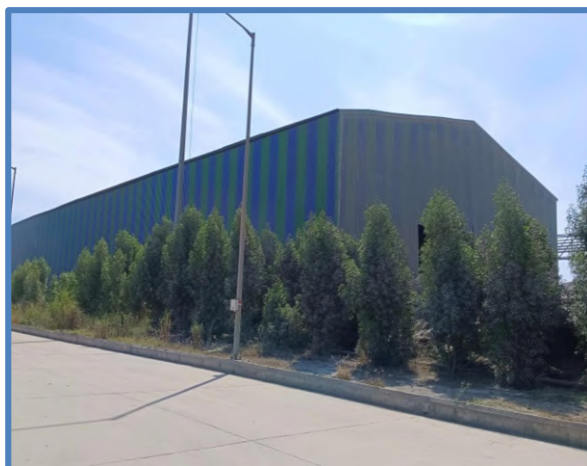
Gypsum storage shed – 5,000 MT
