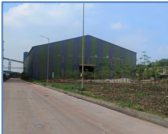
Additive Storage Shed – 10,000 MT
