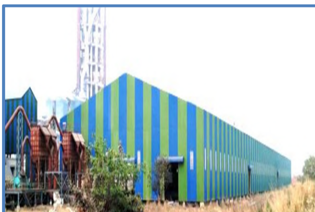
Coal Storage Shed - 20,000 MT
