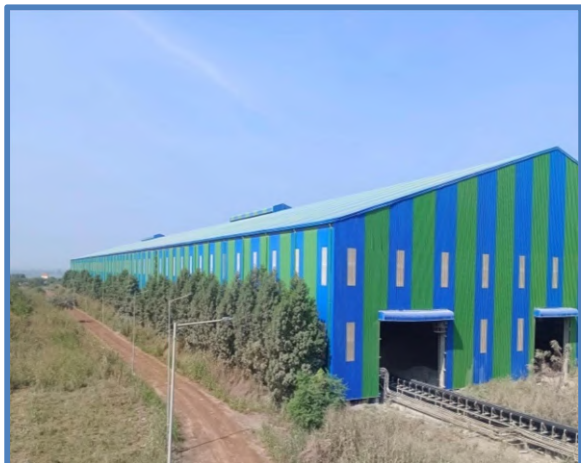
Limestone Storage Shed - 1,00,000 MT
