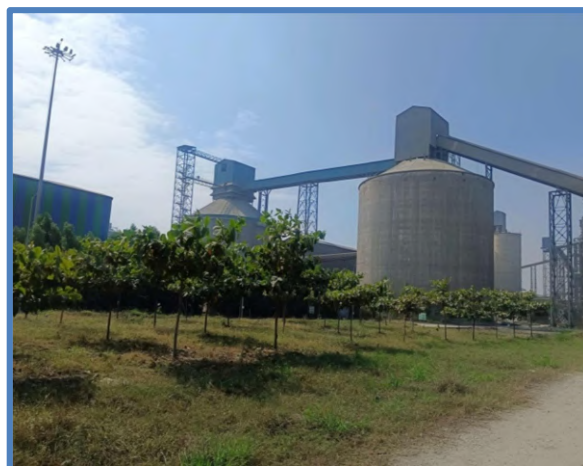
Silo for Clinker Storage – 2 X 50,000 MT
