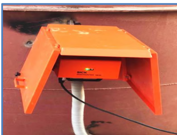
PM CEMS for Coal Mill Bag House Stack
