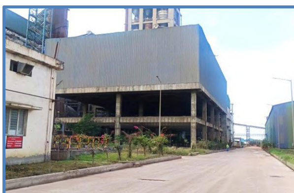
Air Cooler Condensers (ACC)
