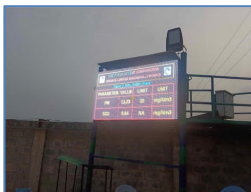
Displaying of Stack emission
