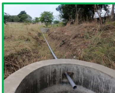
Admin Building Area
