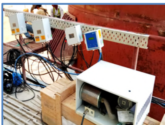
PM & Gaseous CEMS for Kiln & Raw Mill RABH Stack
