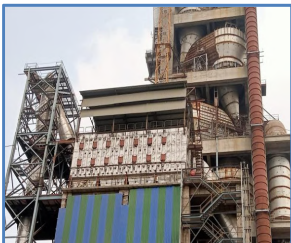
Bag House for Coal Mill
