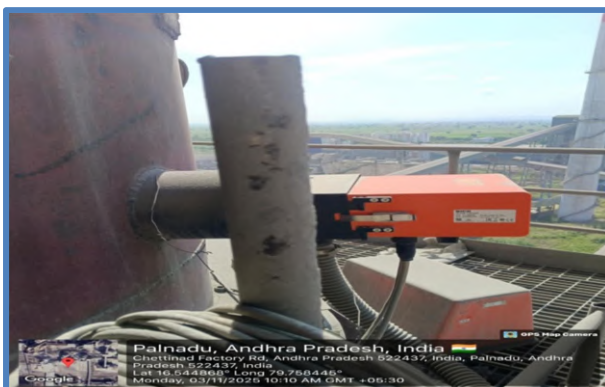
PM CEMS for Cement Mill Bag House Stack
