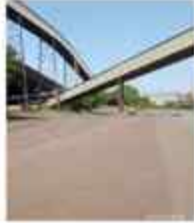
Coal tippler Ramp Entrance Before
