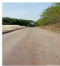
Gypsum yard road Before
